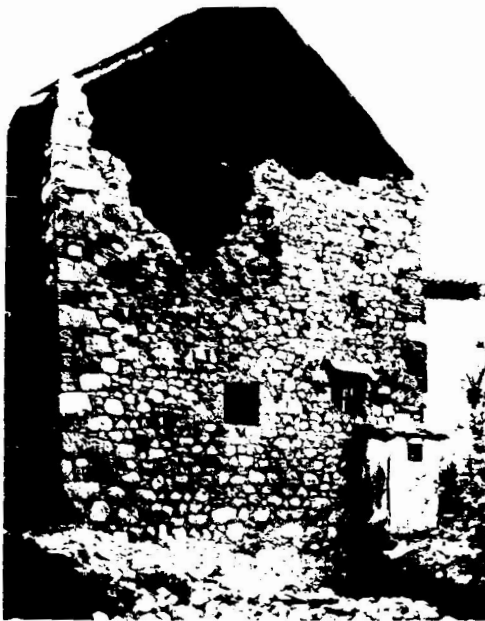
Fig 1. Typical partial collapse of a gable and disintegration of walls of a traditional stone-masonry house
